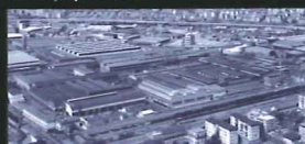
Bolzano plant, ITALY
